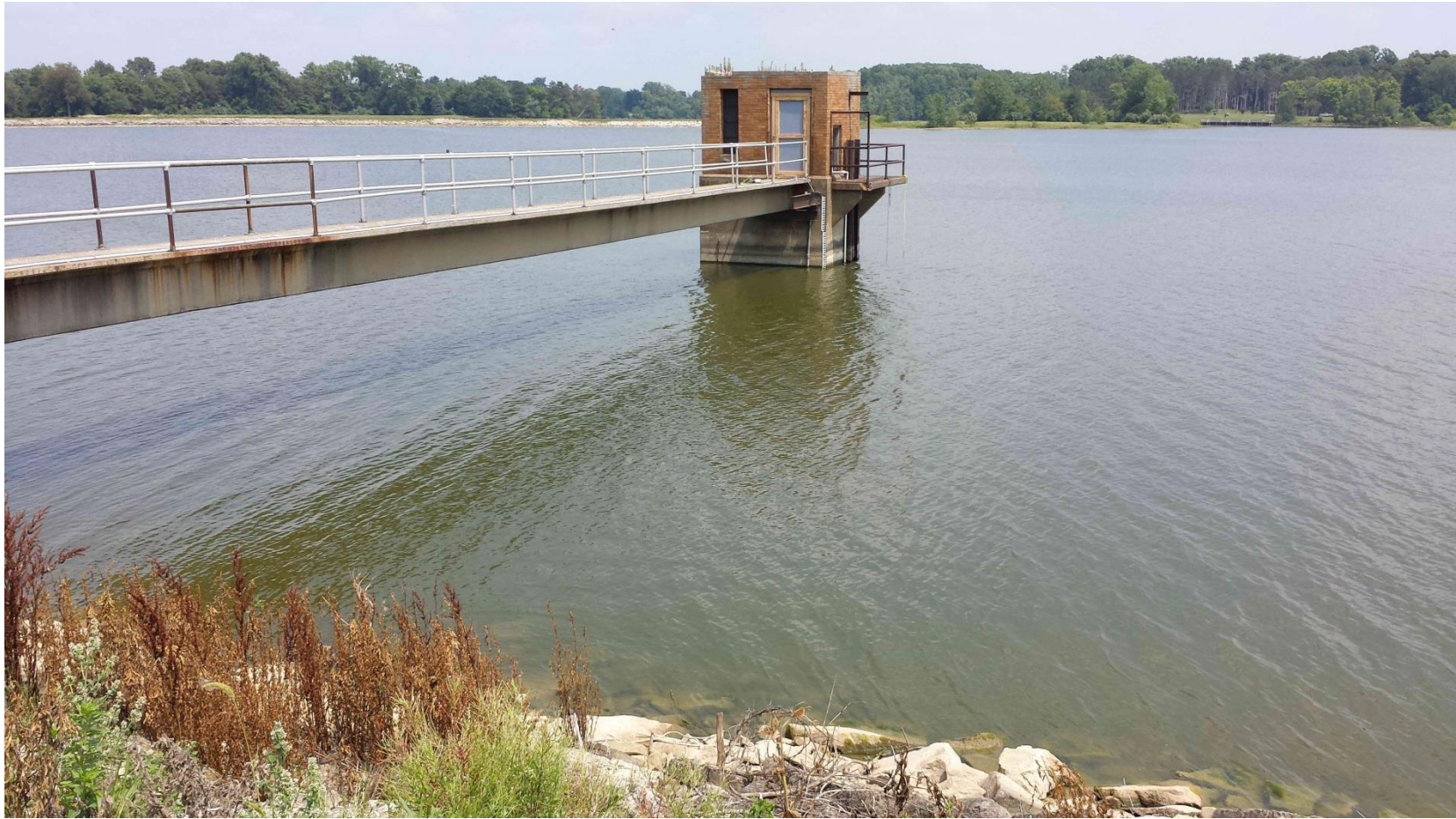
Intake structure for transfer from Middle reservoir to Lower Reservoir
